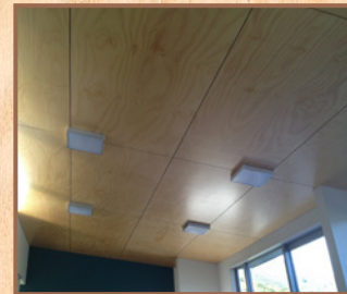
Hoop Pine is the Australian that's winning Kiwi hearts. Left: Elegant bathroom interior, Auckland. Above: Ceiling, South Canterbury.
